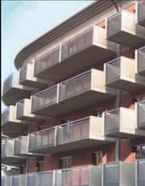
Mesh: Fils 21 - Hot dip galvanised carbon steel
