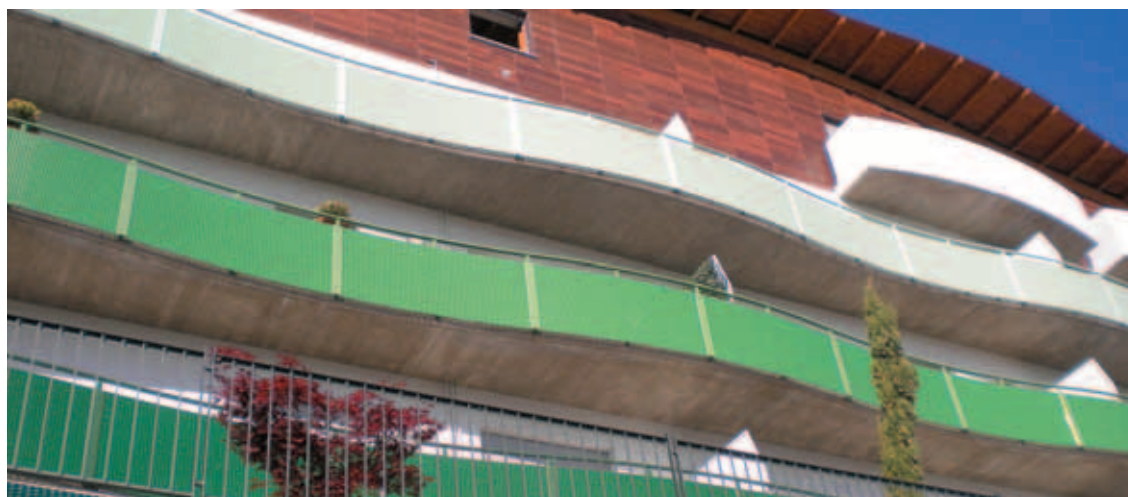
Project: Ing. Giuditta Pezzotta - Mesh: Idea - DL 76 x DC 31 (24) - av 11 x sp 1.5 mm Painted galvanised carbon steel
