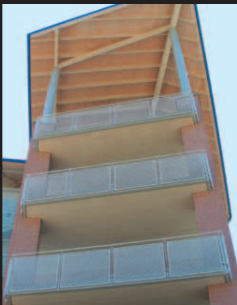
Mesh: Esperia - Hot dip galvanised carbon steel
