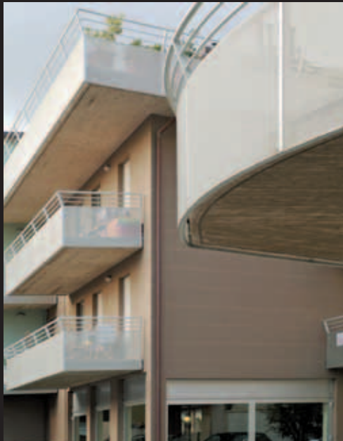
Mesh: Perforated sheet metal - Round hole
