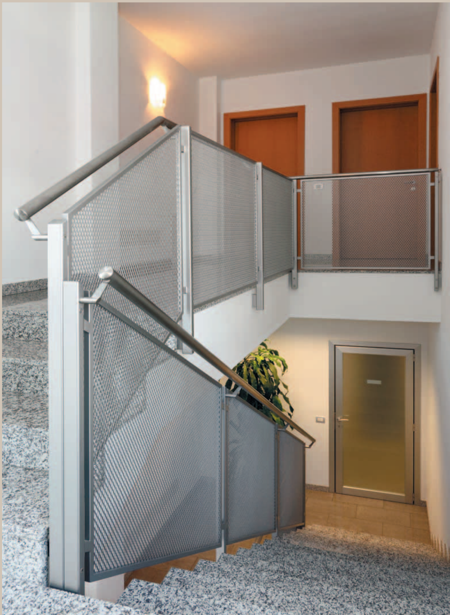
Mesh: DL 28 x DC 16 - av 3 x sp 2 mm - Painted Sendzimir carbon steel Photo: Studio Diecidodici
