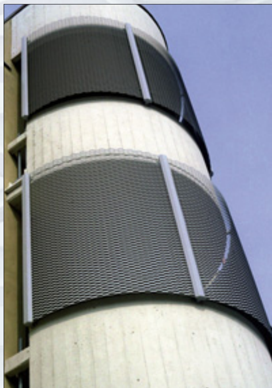
ESPERIA - DL 100 x DC 40 (34) - av 15 x sp 1.5 mm Aluminium painted with polyester powder exterior paint
